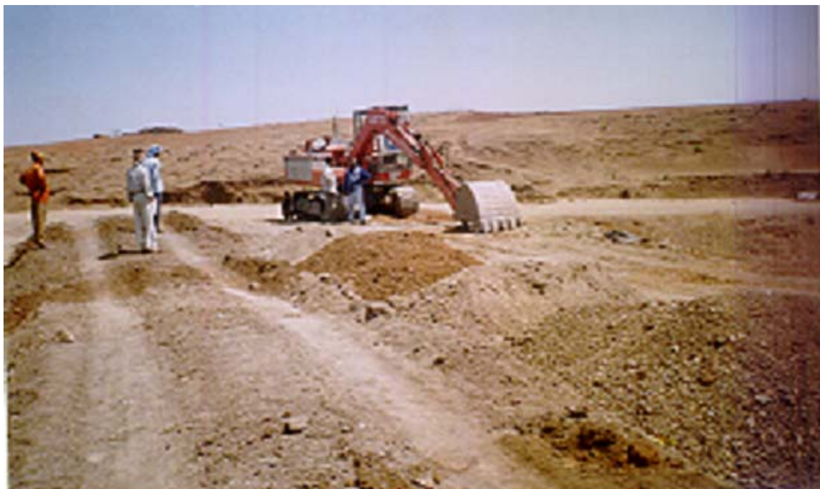
EXCAVATOR IN OPERATION AT RELIEF SITE Village: LANGDI MOHADI, BARWANI DISTT., M.P.
